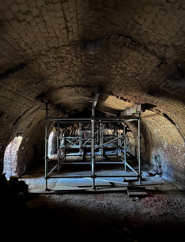
Figure 5: Temporary stabilisation works to reduce further collapse of kilns
